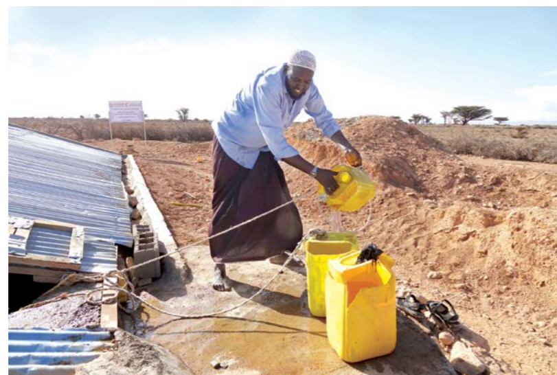
Water tank in Boocada
